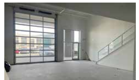
Inside view (top) and parking lot facing view (bottom) of #3 – 6676 152nd Street. PHOTOS Courtesy of Kelly Bowman
